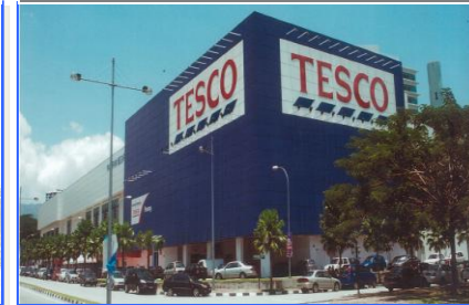
TESCO Building Penang
