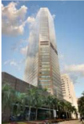
Six Battery Road
